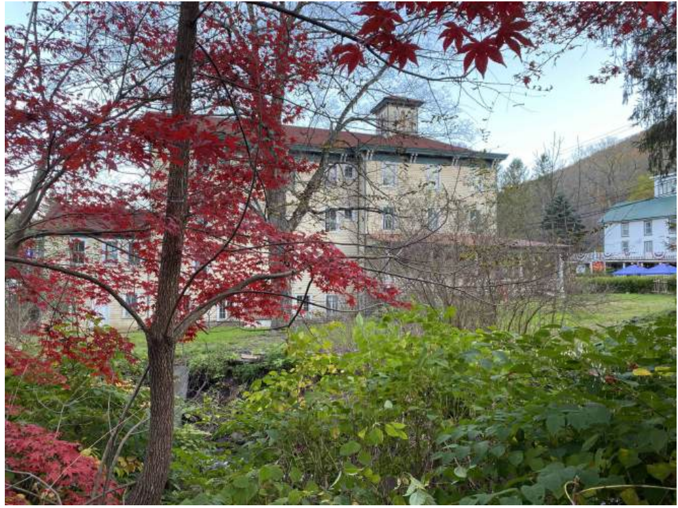
F6 L003 SITE PHOTO 1 - JAPANESE MAPLE TO REMAIN, VIEW EAST FROM CREEK NOT TO SCALE
