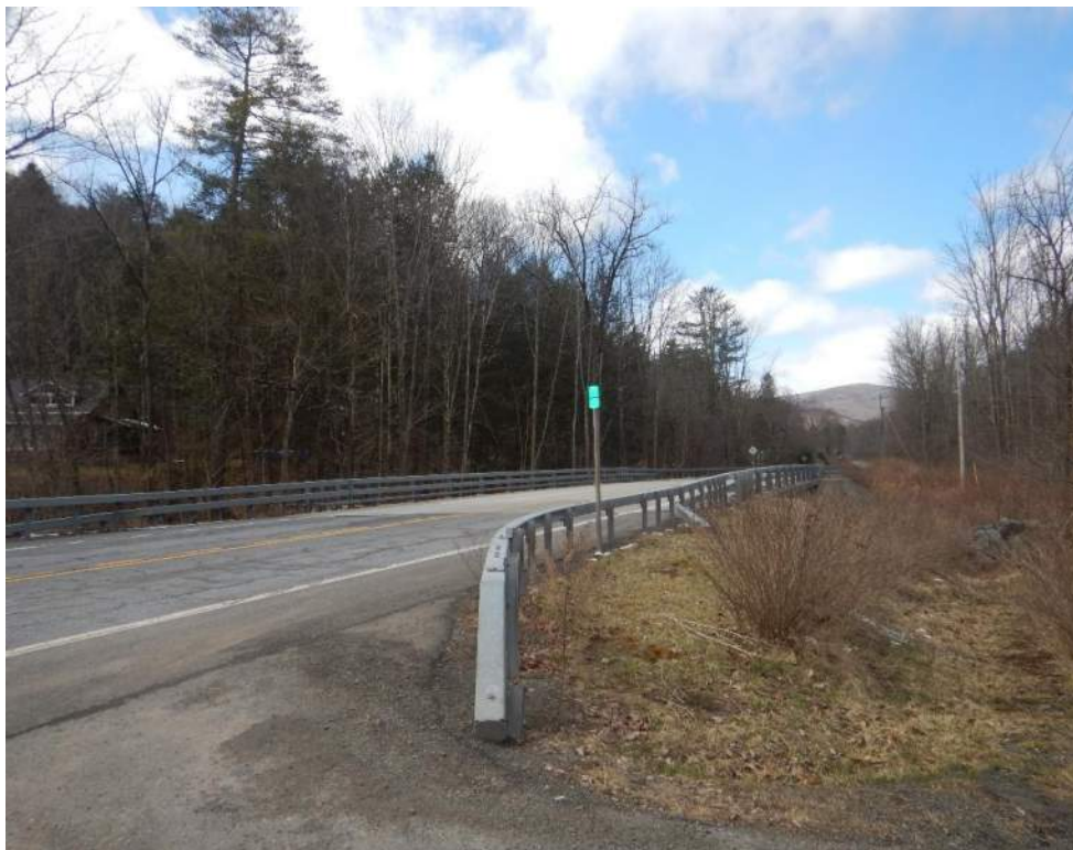
Photo 13: Poor sight distance onto Route 42 due to bridge guiderail, looking north.
