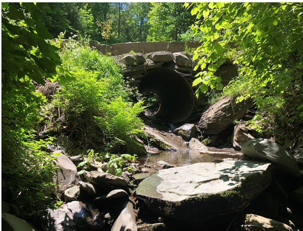
Figure 4-44: Outlet and tailwater of Station Road culvert at Woodchuck Hollow
