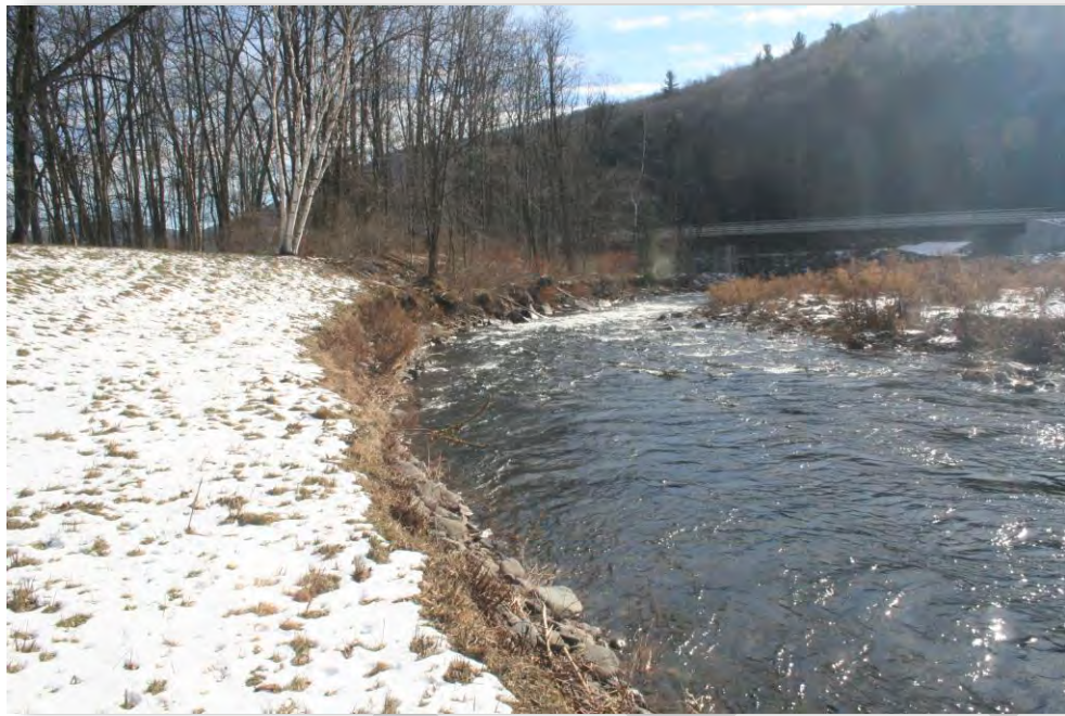
Figure 2-8 Erosion along Flood Control Levee in Shandaken
